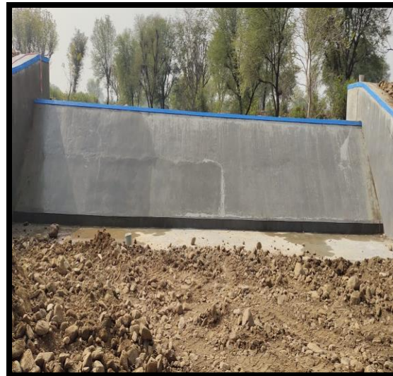
Kundwari wala Check Dam
