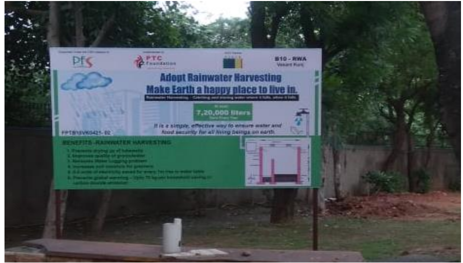
Rain Water Harvesting Structure- B 10 Vasant Kunj
