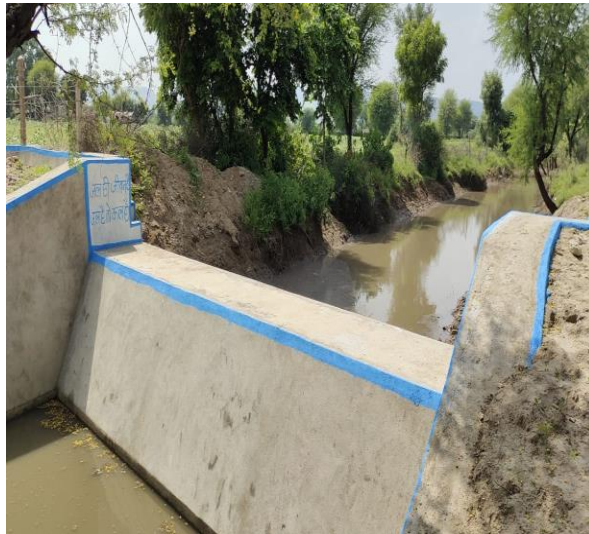
Peel Wala check Dam
